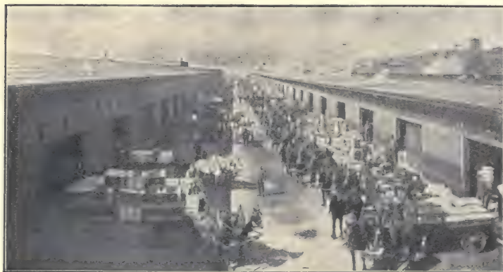
FIG. 109—Grand Trunk Freight Sheds, Toronto, Ont.
